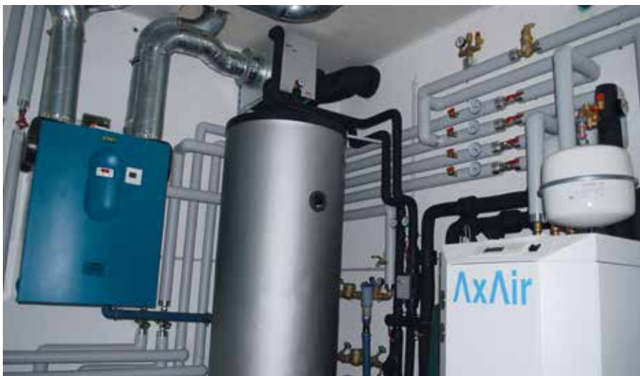
Fig. 24 | The power house with heat pump, hot water boiler, circulation pump and distribution lines, etc. is assembled manageably in the smallest possible space.
