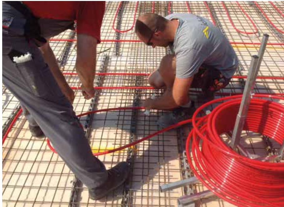
Fig. 3 | The installation of heating and cooling registers into the ceiling can be done quickly, easily and therefore economically. © Aichinger Hoch- u. Tiefbau GmbH
