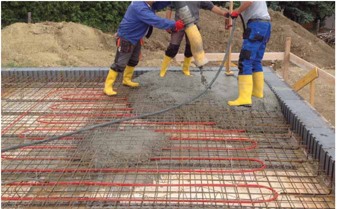
Fig. 1 | During component activation, a system of water-conducting pipelines is laid into concrete components. This is perfectly easy to accomplish. © Aichinger Hoch- u. Tiefbau GmbH
