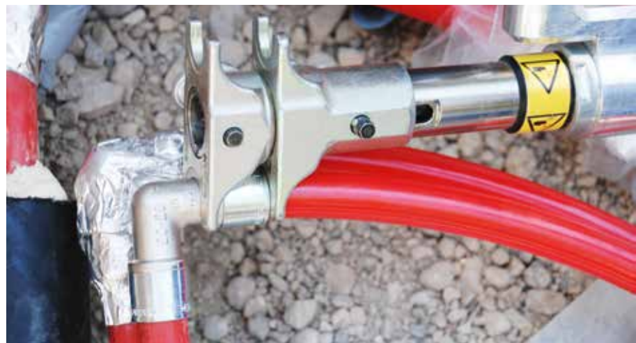
Fig. 42 | When dividing up pipelines, a sleeve is slipped onto the coupling with a press and then shielded. © Rehau
