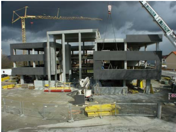
Abb. 6: Montage Sandwichwand
