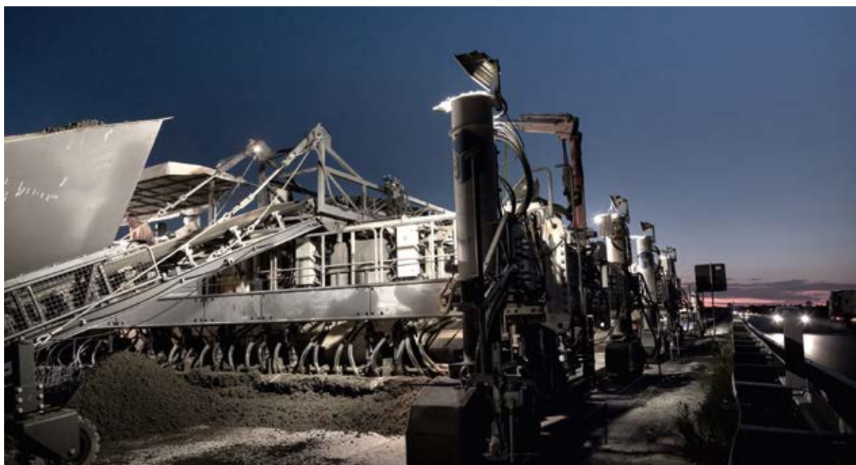
Betonfertiger in Action
